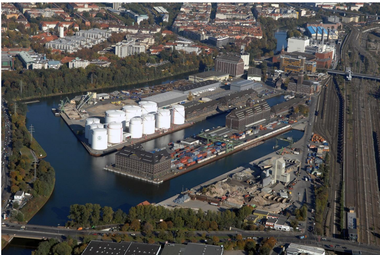
Aerial photo Westhafen Berlin (Source: www.euroluftbild.de )
