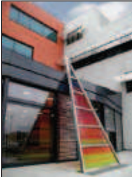
Architectural elements for recooling
